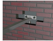
Installation of the re-usable wall tie
