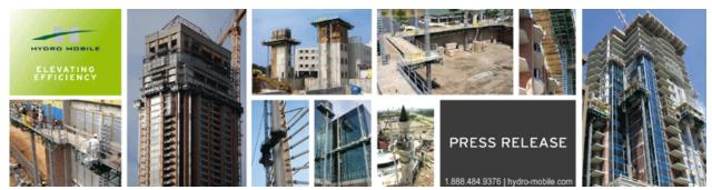
used to access the most restricted locations. Four F-Series were used for their versatility and because they can operate in split mode, which allowed Limen Group to bring one side down to load material while the other side stayed above the church's roof.
